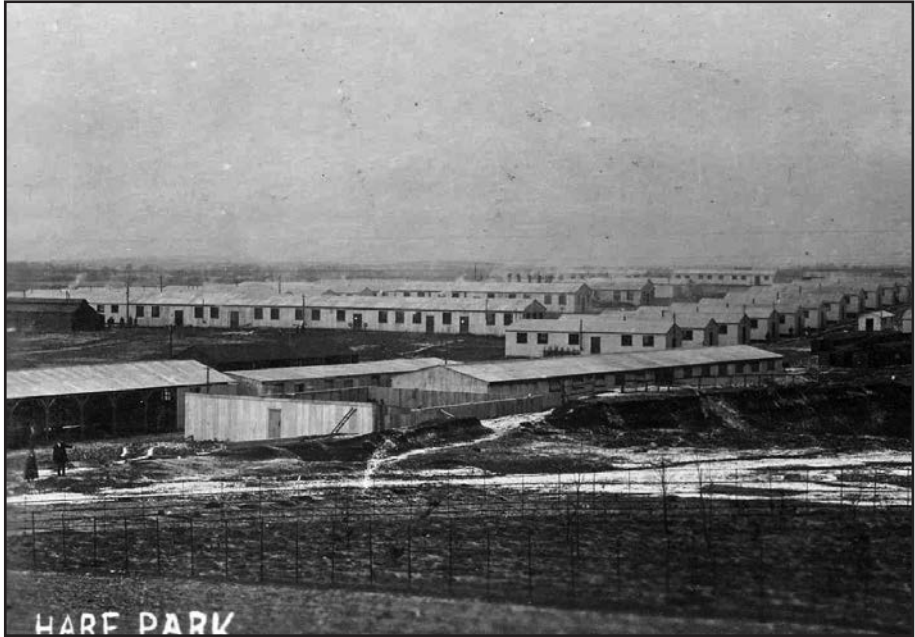
Hare Park Camp, the Curragh, under construction.
